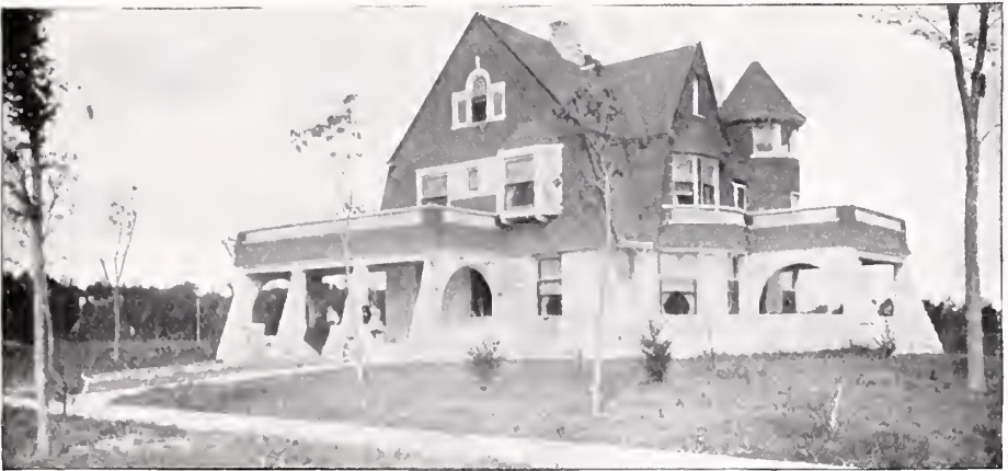
RESIDENCE OF F. P. BURNHAM, FIRM OF EDBROOKE & BURNHAM, ARCHITECTS, CHICAGO, ILL.
